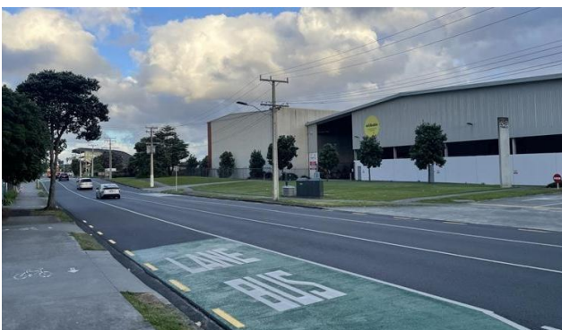
Figure 3: Puhinui Rd bus lanes. (Source: James Wratt)
