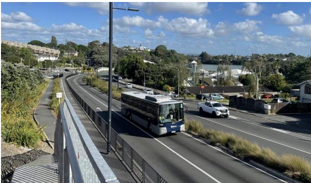
Figure 2: Eastern busway. (Source: James Wratt)
