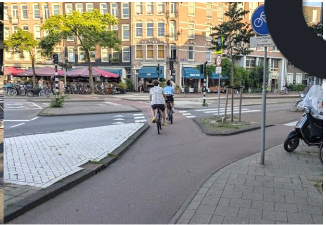
A protected cycle roundabout in Amsterdam
