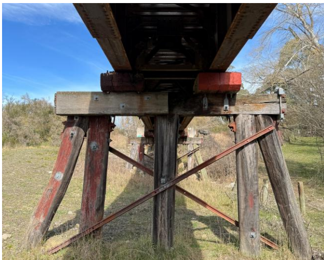
Before: old bridge piers
