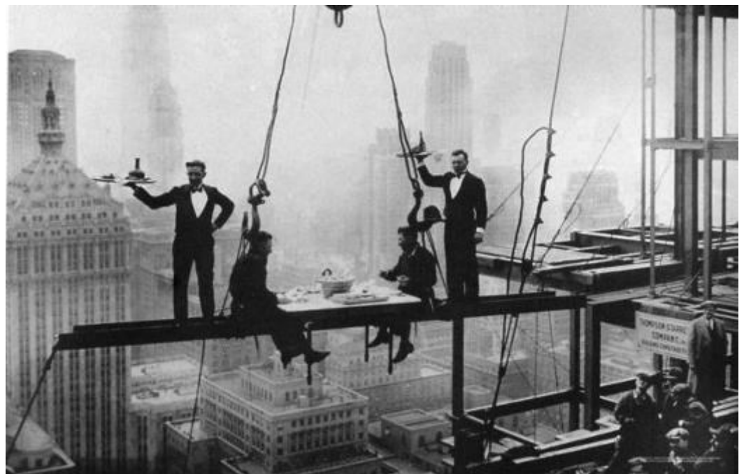
Waiters serve steel workers lunch on a girder high above the Waldorf-Astoria Hotel, New York, 1930
