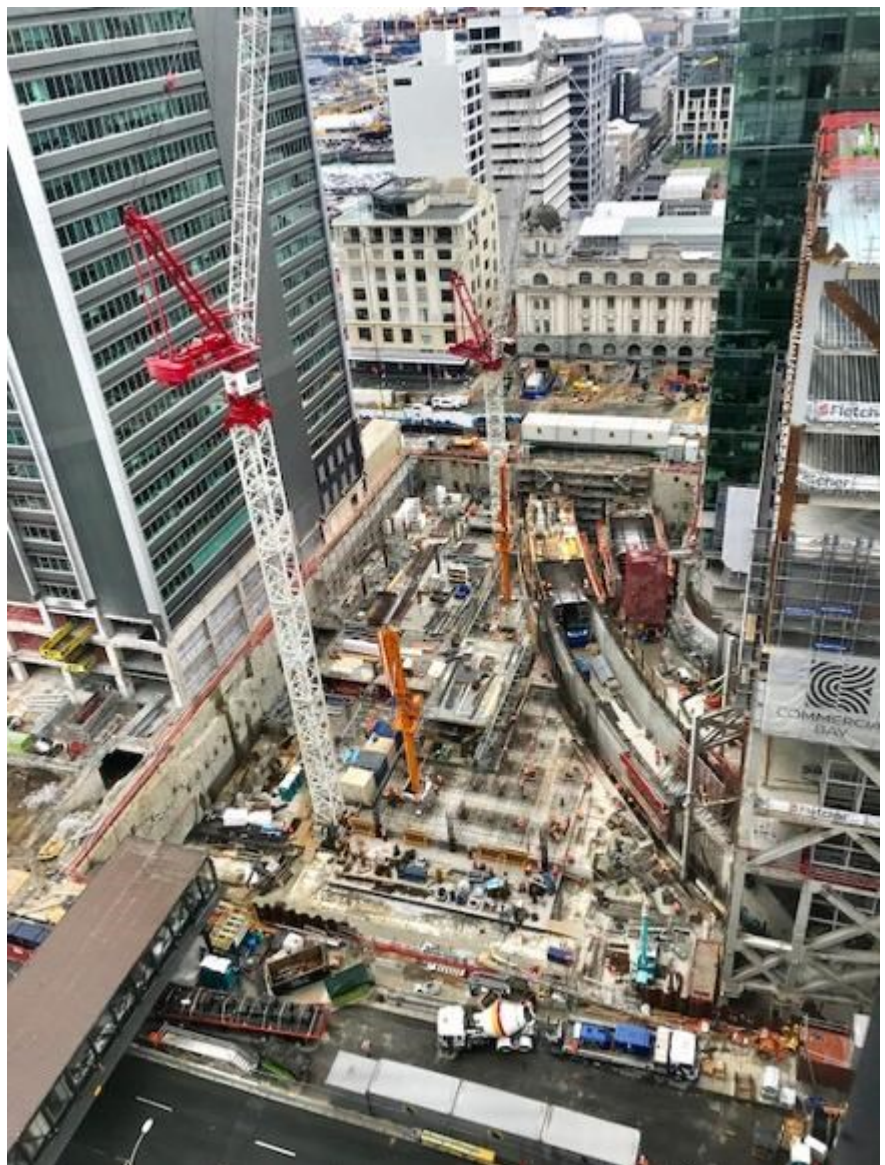
Image from 2019 showing the curving rail tunnels emerging from under the CPO and through the basement of what was to become the Commercial Bay tower
