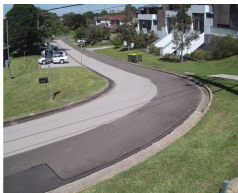
Half of this residential street in Parramatta is covered with a paint that reflects solar radiation, keeping it at least 10C cooler than the untreated section on a normal summer's day.
