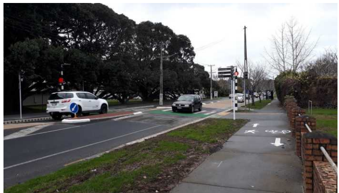
Figure 8: Carrington Rd crossing after implementing the raised paired crossing
