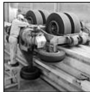
Figure 13: ALWEG running gear
