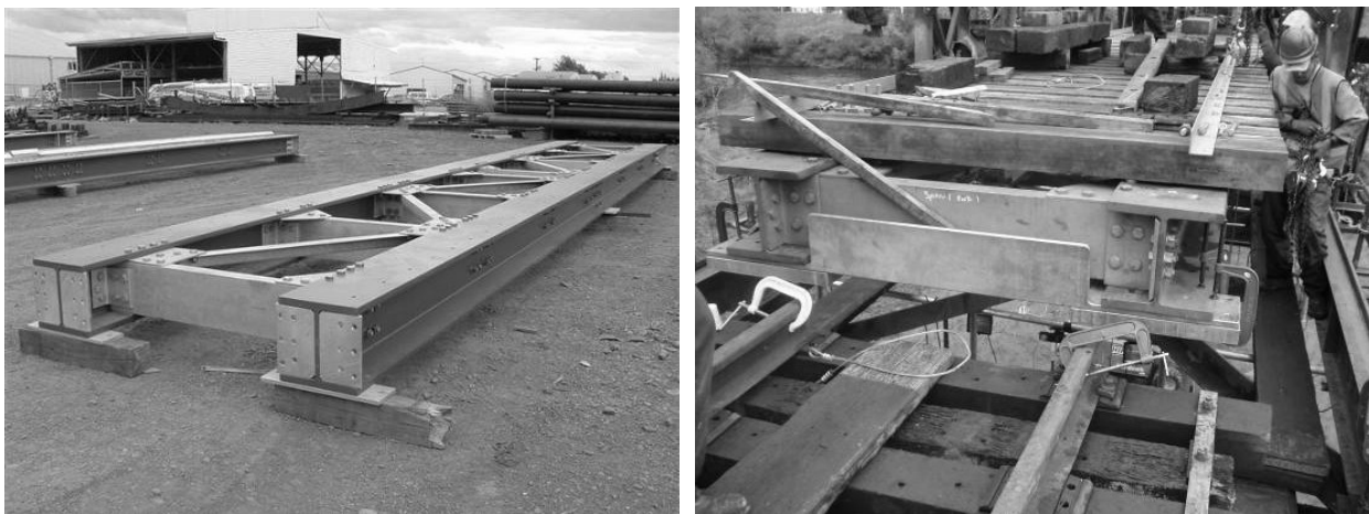
Figure 3.4 – Left: example of a standard steel 'I' beam unit after fabrication. Right: a TSEP unit complete with sleepers installed being lowered into place on a bridge.
