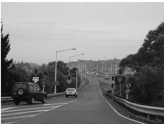
Figure 16: Photos of the Easy Merge Ramp Signal in operation
