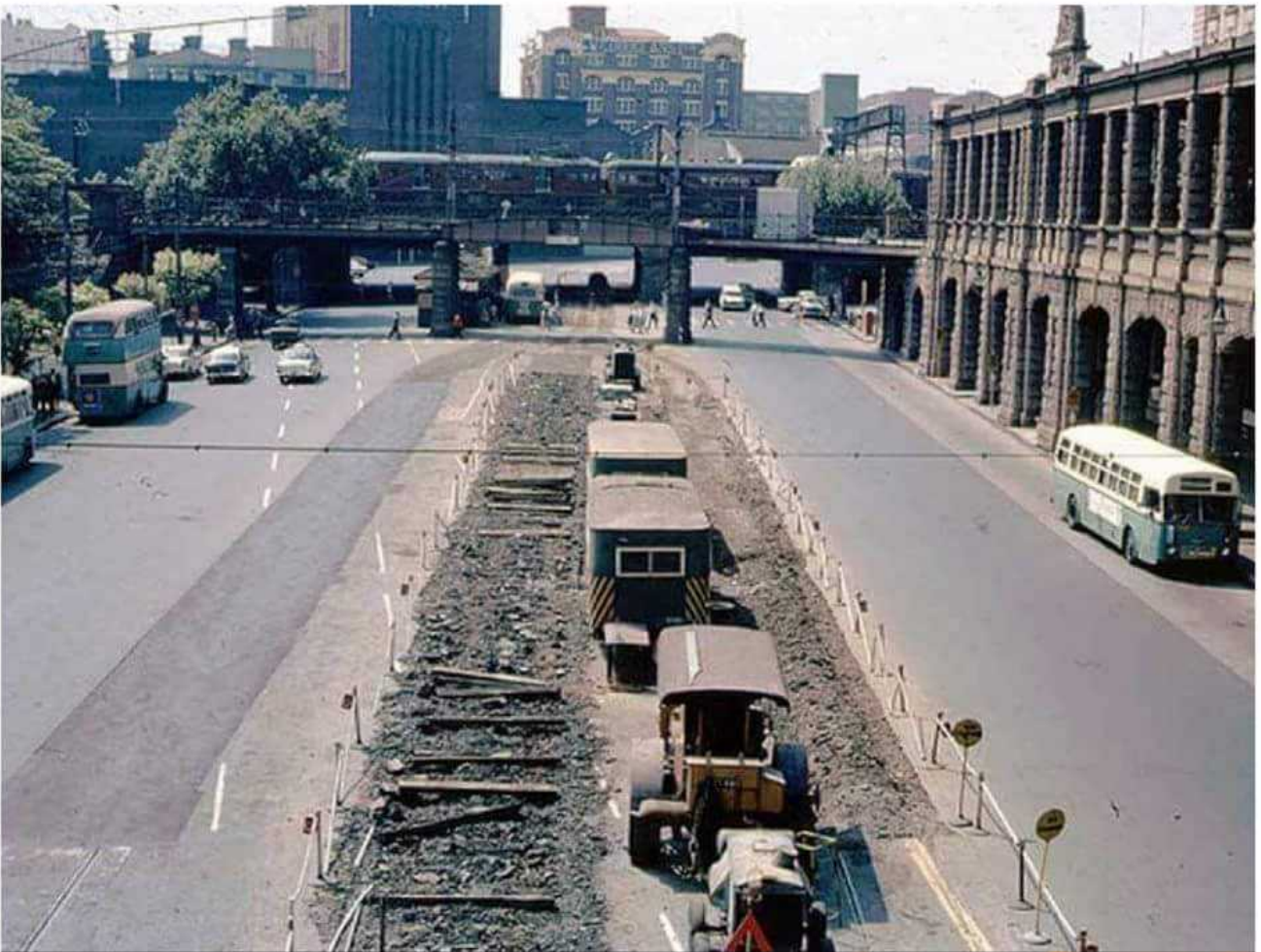
Sydney tram tracks being removed in the 60s... And being put back in in 2017.
