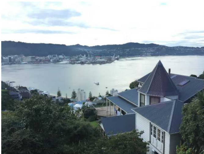
View overlooking the Port of Wellington, with earthquake damage visible from across the bay
