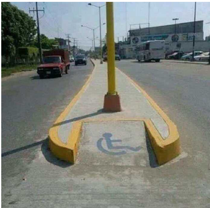
Something about this ramp seems to make it less useful for wheelchair users...
