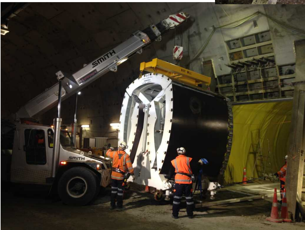
Above: 20t crane lifting the arm form onto the steel track
