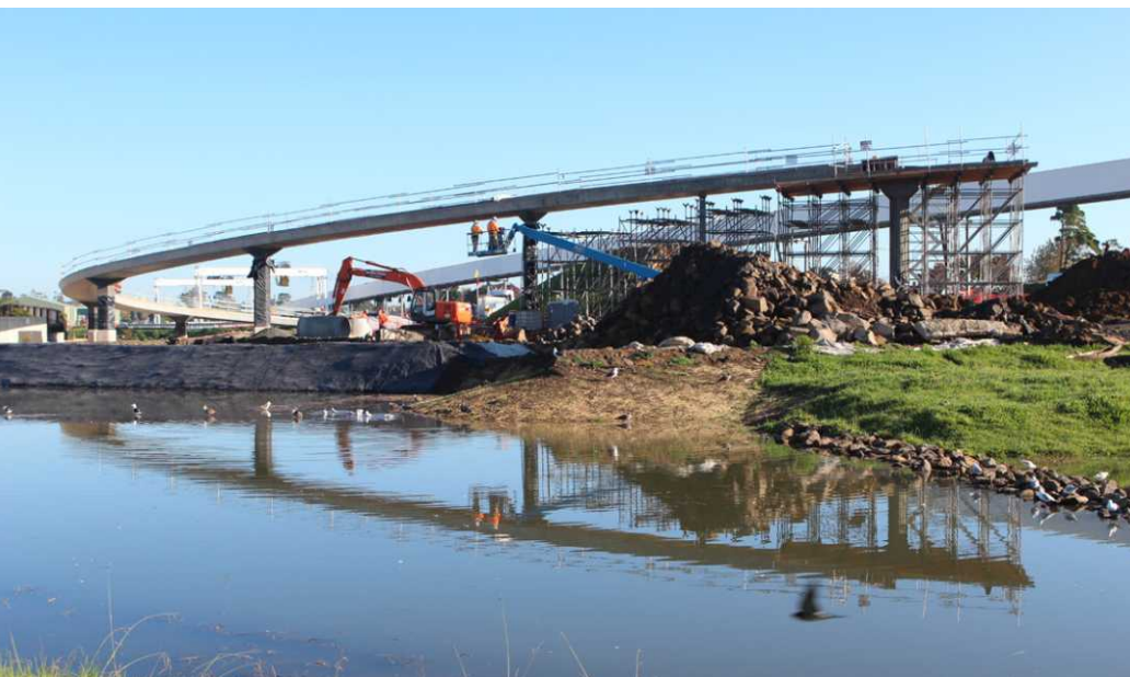
The Hendon Footbridge under construction
