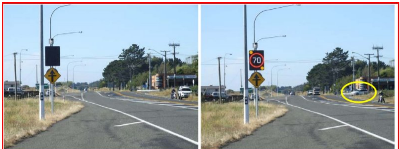
Figure 3: The RIAWS in operation at Himitungi with no conflict risk (left) and a potential conflict risk (right) with a side road vehicle present (circled)
