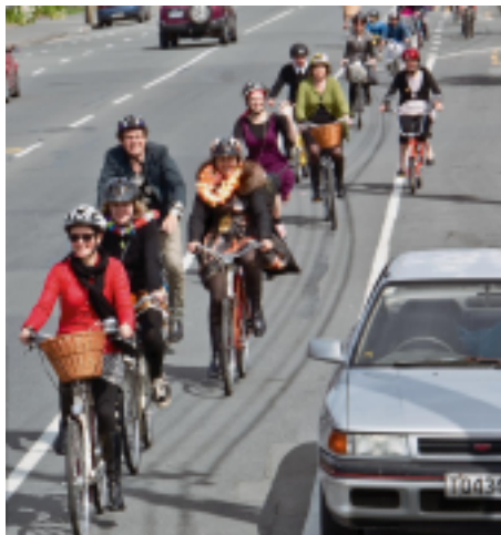
A well-designed cycle lane with plenty of door-zone clearance (Christchurch)
