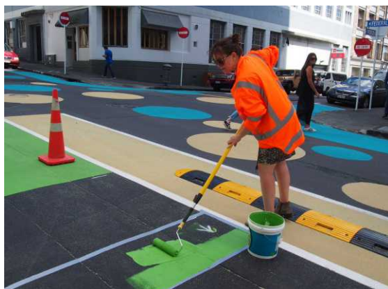
Associate Minister of Transport Julie-Anne Genter helps install the contra-flow cycleway on Federal St
